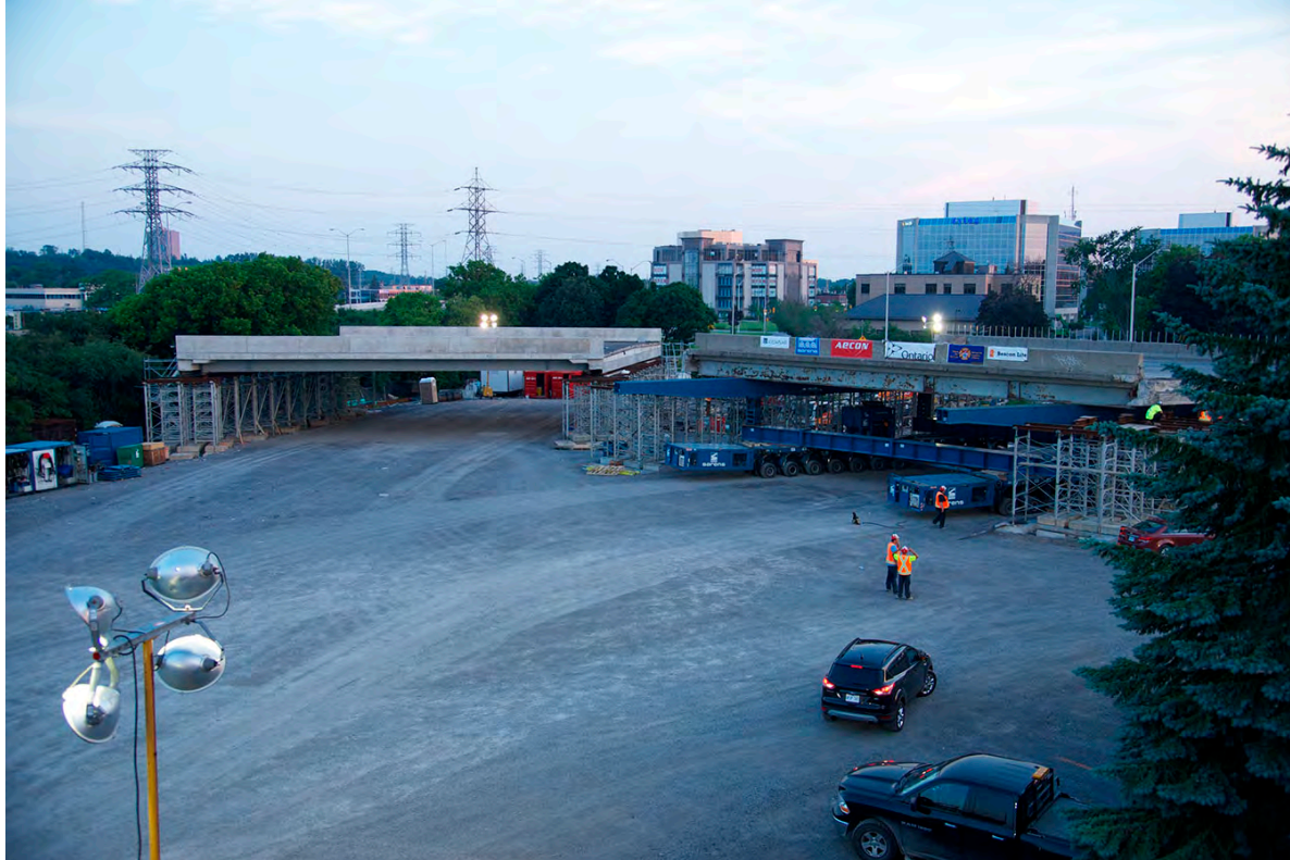
Self Propelled Modular Transporter (SPMT) - exchanging old deck and girders for new.
