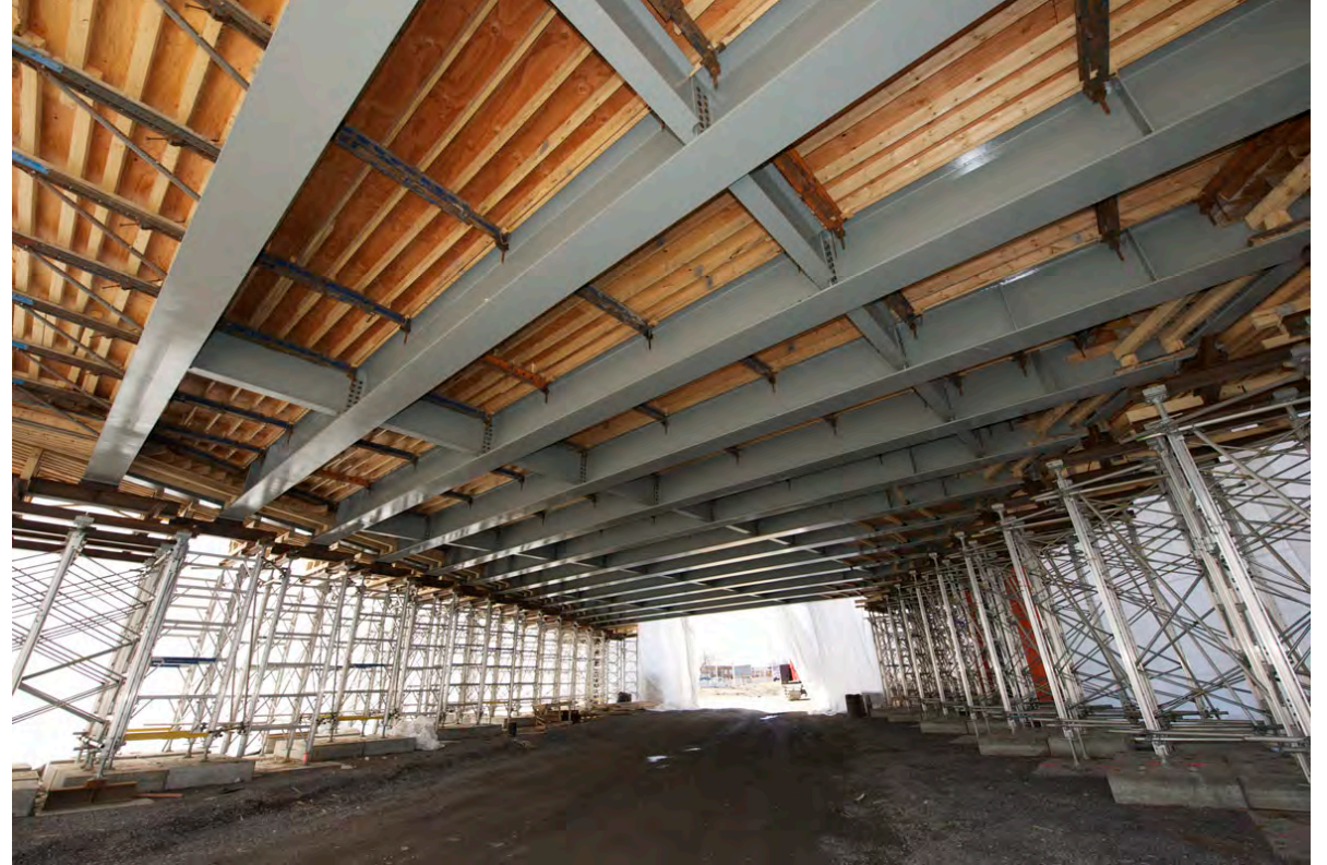
Temporary support structures in staging areas.
