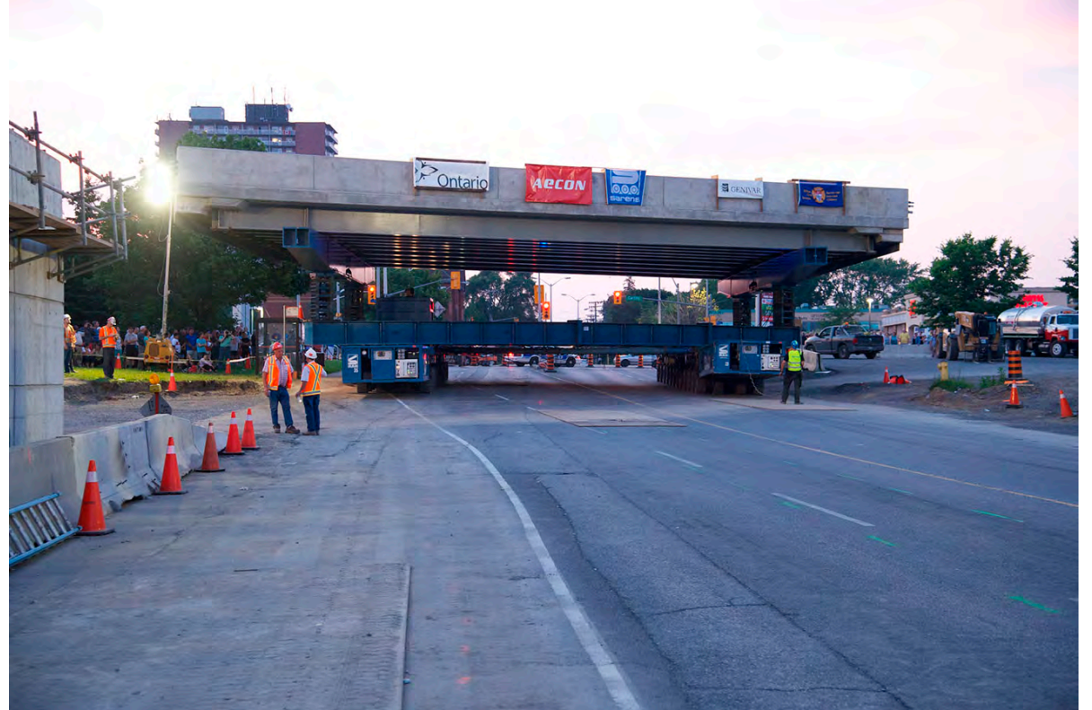
SPMT - delivering new deck and girders for placement on substructure.
