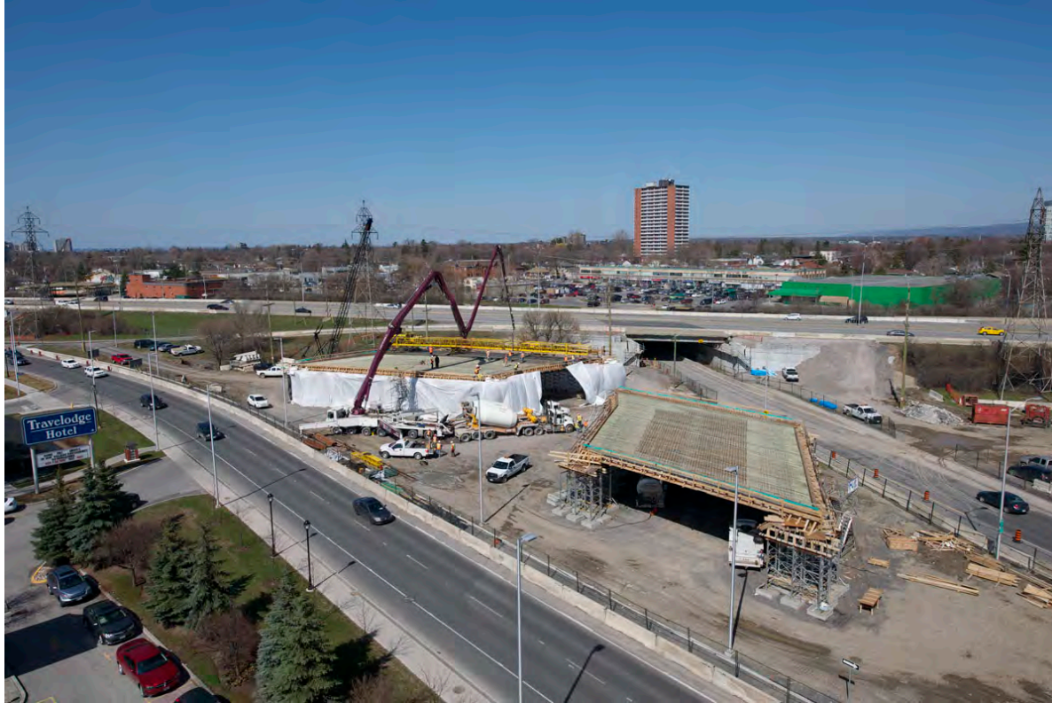
Construction of new deck in staging areas.
